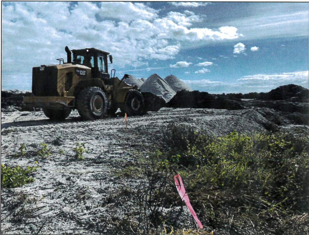
DMMA Settling non-beach compatible material staged for removal 12-3-20
