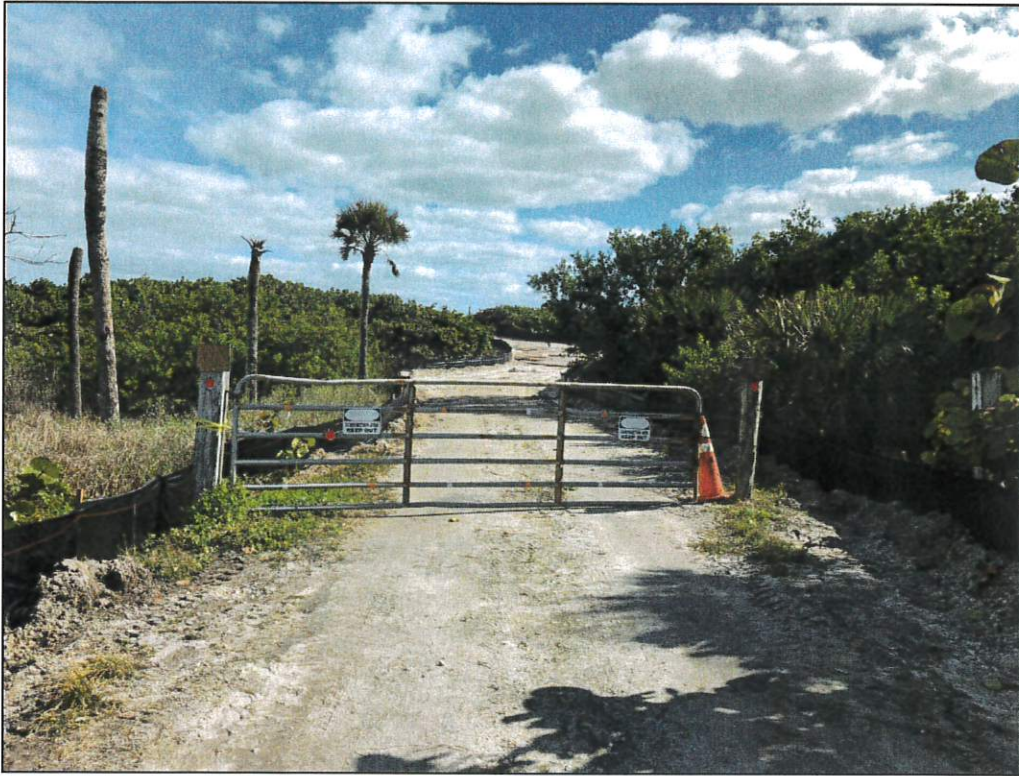
R-8 beach access preparation for project – 12-3-20
