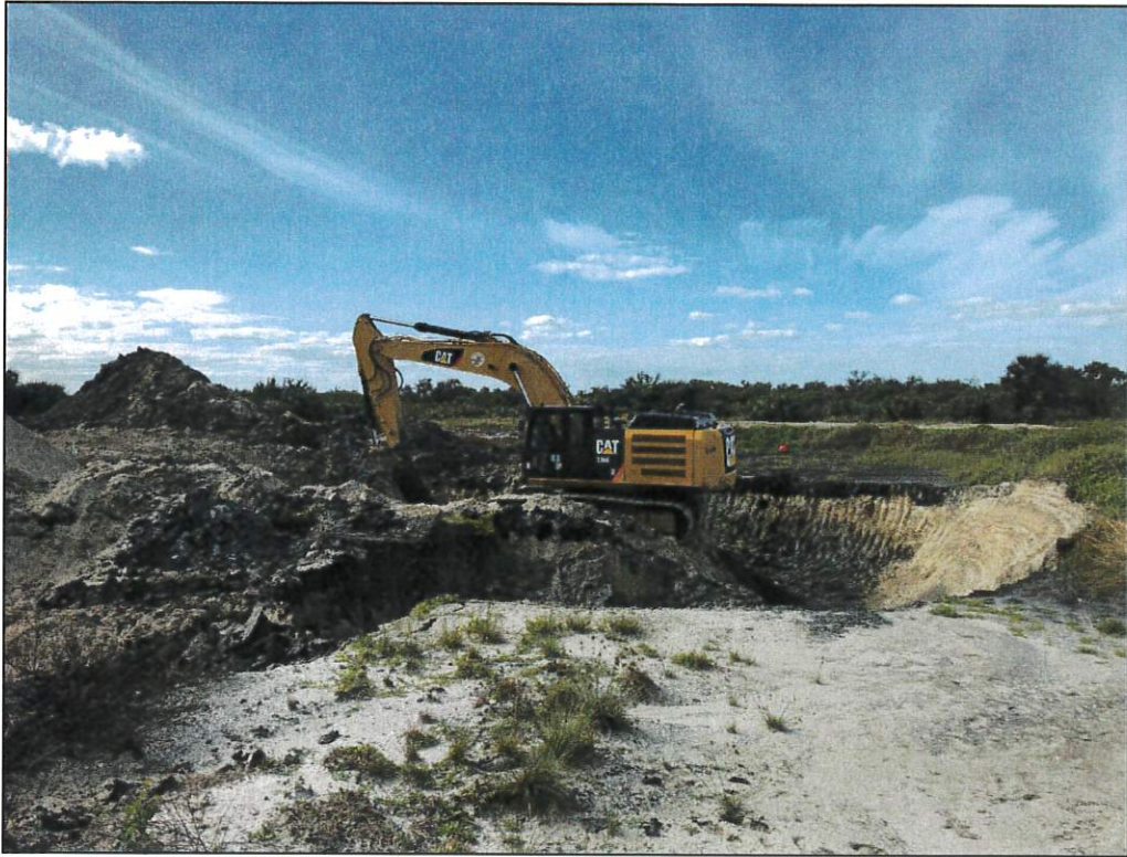
DMMA Settling Basin Excavation of non-beach compatible material 12-3-20
