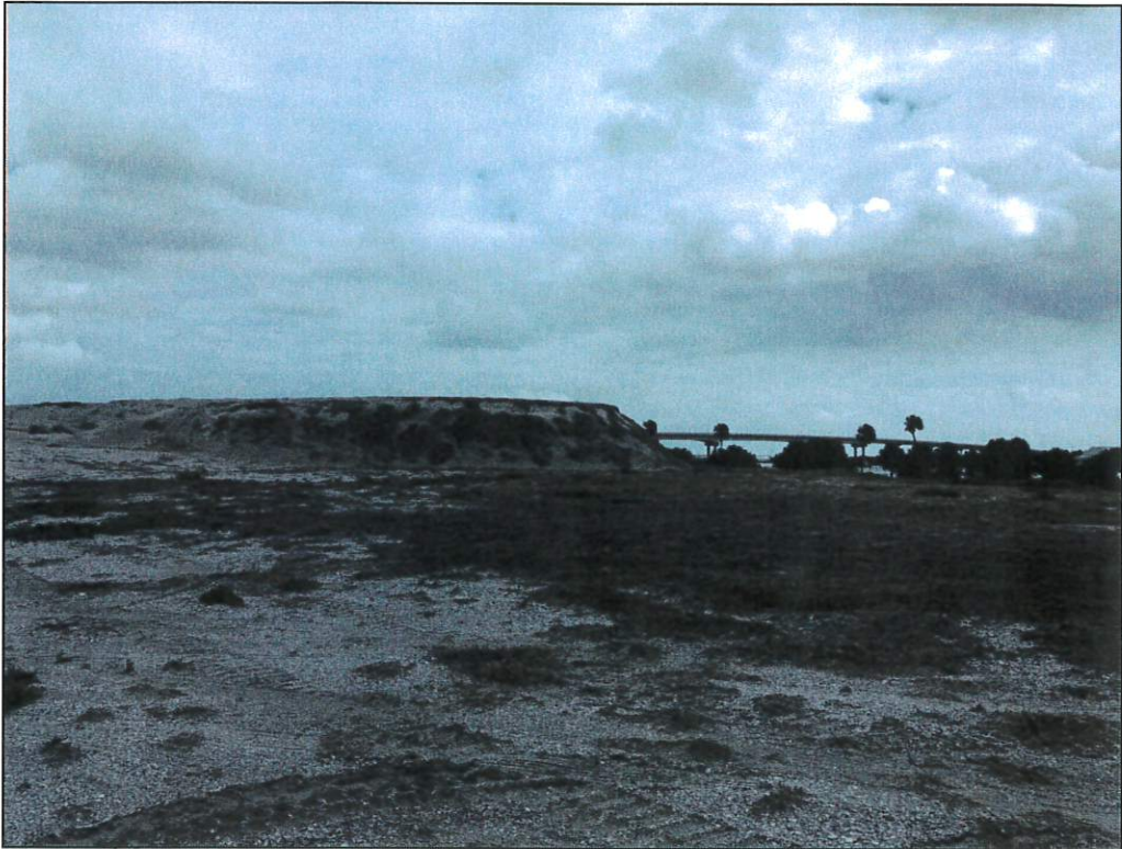
DMMA Pre-Construction Activities looking Northeast – 11-19-20
