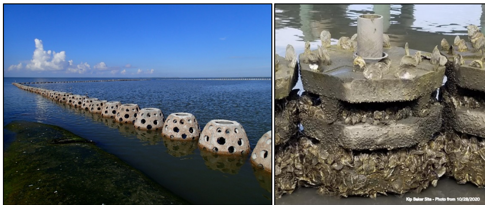
Figure 5-1. Example of concrete cast oyster products – Reef Innovations Reef Balls (left); Reef Maker Wave Attenuator (right).
