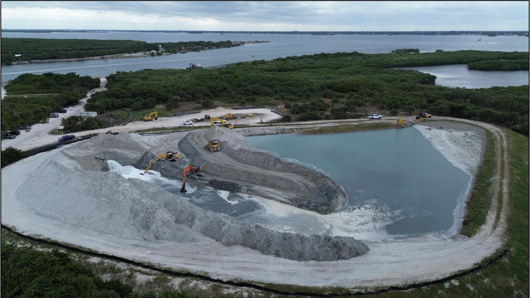
Figure 7. Aerial photo of material being pumped from Sebastian inlet complex into the Dredged Material Management Area (DMMA). The DMMA is within the Sebastian Inlet State Park and managed by the Sebastian Inlet District to conduct sand bypassing activities southward along the beaches of Indian River County. Photo was taken by ATL Diversified, Inc. on January 2026, courtesy of James Gray. See additional construction photos of inlet sand bypassing projects.
