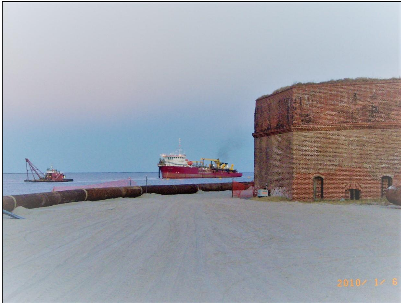
Figure 1. St. Marys River Entrance inlet channel being dredged by the USACE to bypass material south to be placed on Ft. Clinch State Park shoreline. Photo taken by DEP staff. See additional construction photos of inlet sand bypassing projects.
