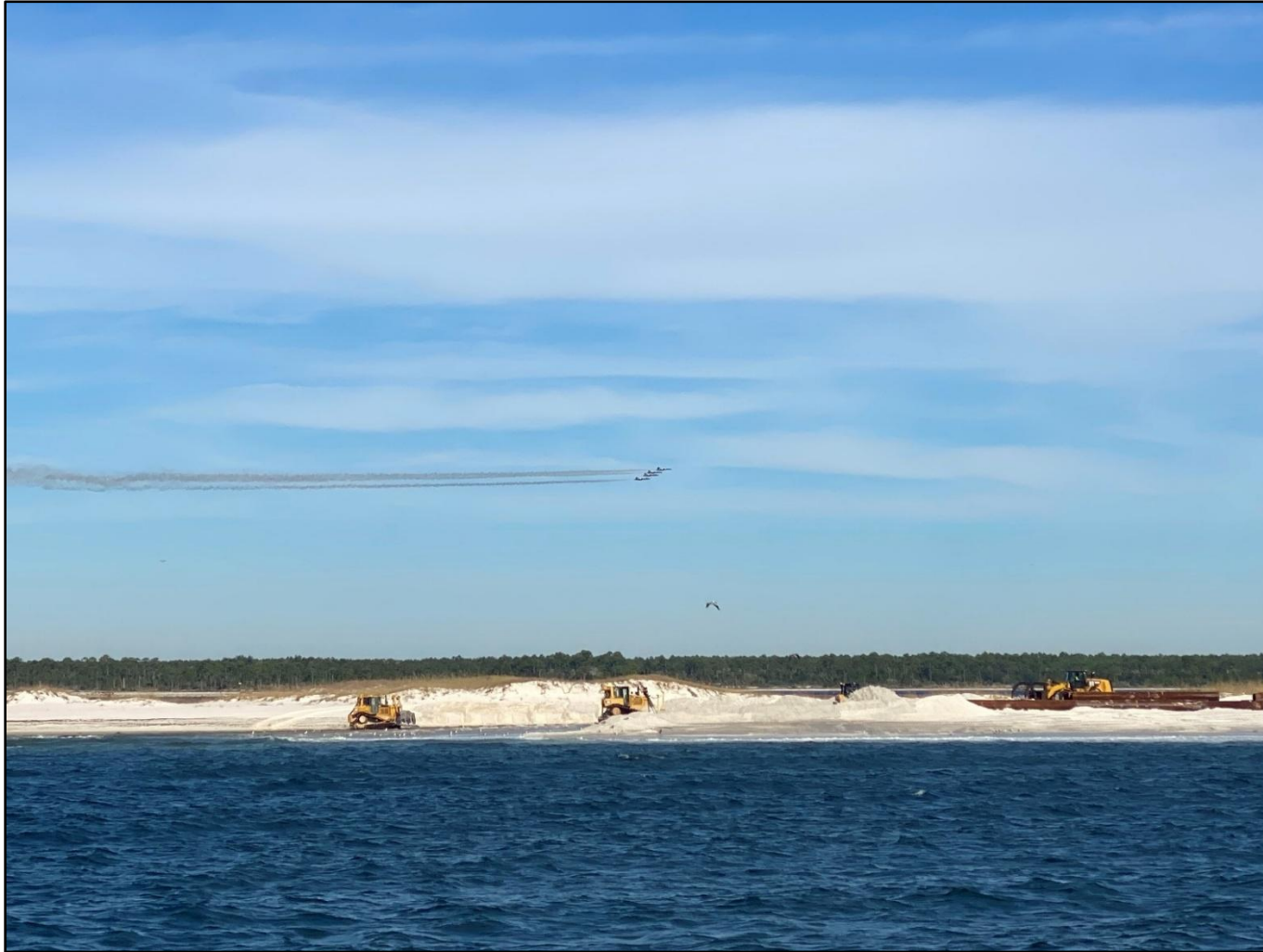
Figure 21. Pensacola Pass Federal Navigation Channel dredged to place material at Johnson Beach in Gulf Islands National Seashore Park on Perdido Key. Photo courtesy of Timothy Day with Escambia County, November 2024. See additional construction photos of inlet sand bypassing projects.
