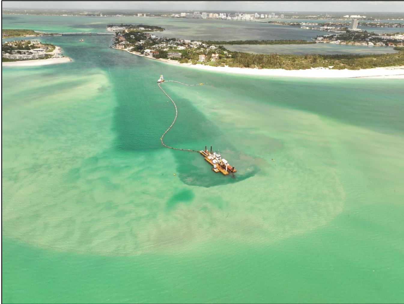
Figure 26. Sand bypassing from the New Pass navigational channel and ebb shoal with material being placed along the Lido Key shoreline. Photo courtesy of Morjana Signorin, P.M., with Coastal Protection Engineering and the City of Sarasota, June 2026. See additional construction photos of inlet sand bypassing projects.
