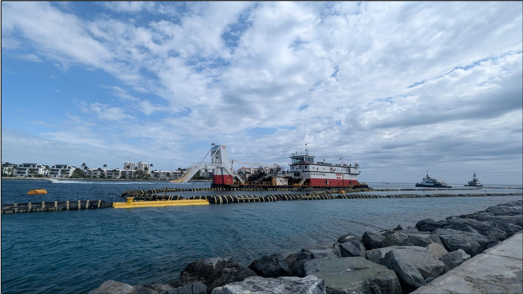
Figure 13. Palm Beach Harbor/Lake Worth Inlet channel being dredged by a Weeks Marine cutter suction dredge to bypass sand south of the inlet to the Mid-Town shoreline. Photo courtesy of the Town of Palm Beach and Sara Gutekunst P.M. The photo was taken in March 2025. See additional construction photos of inlet sand bypassing projects.
