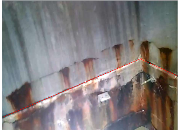
Bay 48 - Looking South
