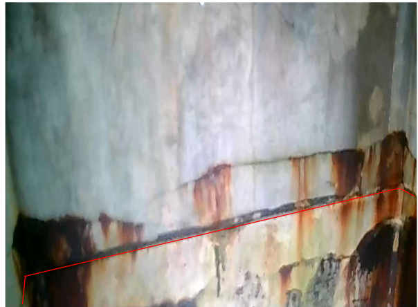
Bay 39 – Looking South
