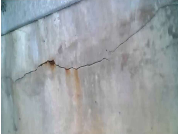
Bay 5 - Looking East
