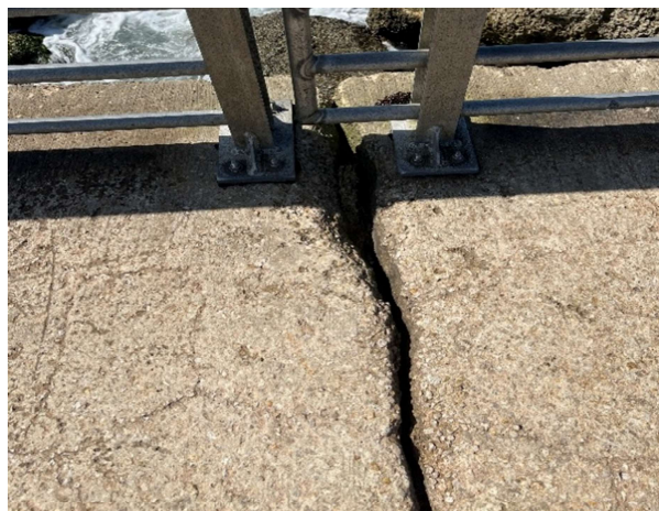
Typical construction joint
