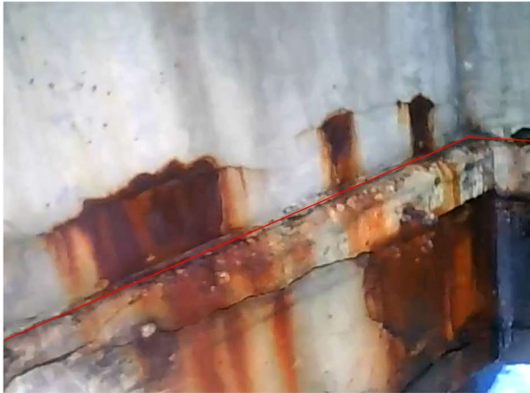
Bay 53 - Looking West
