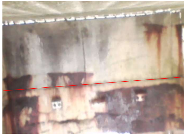
Bay 25 – Looking south
