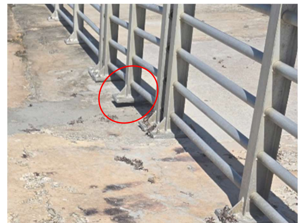
Unsupported intermediate post base plate
