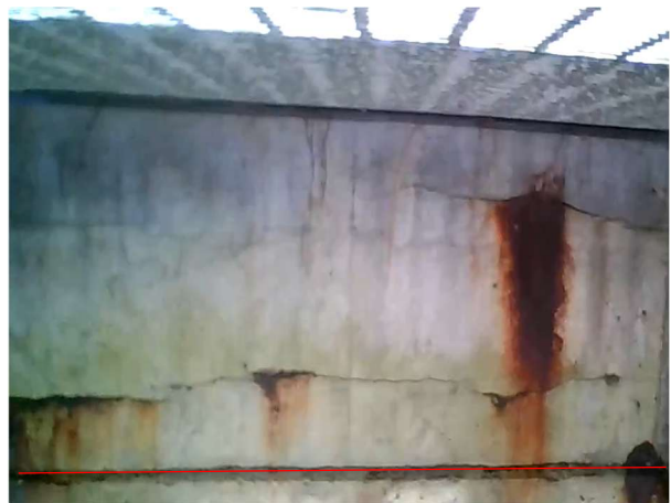
Bay 27 – Looking North
