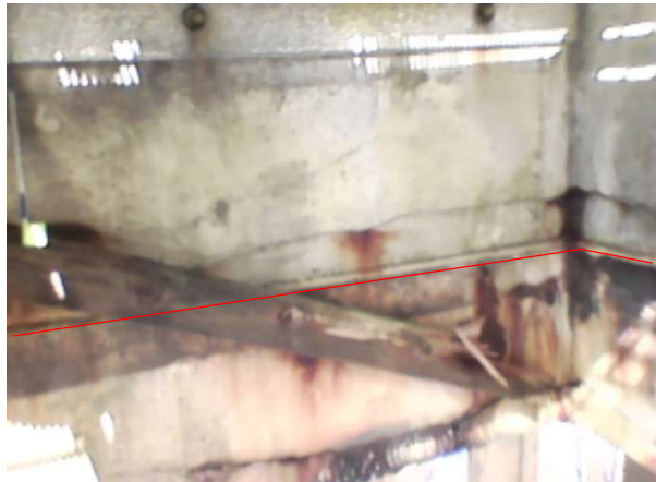
Bay 13 – Looking west
