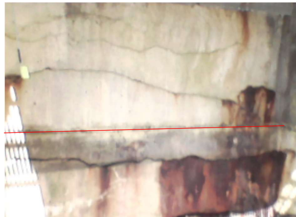
Bay 19 - Looking west
