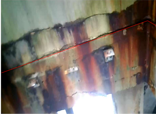
Bay 34 – Looking South
