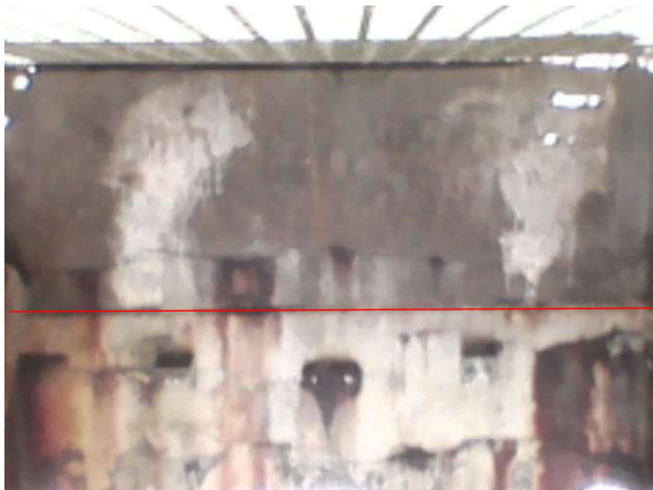
Bay 20 - Looking north
