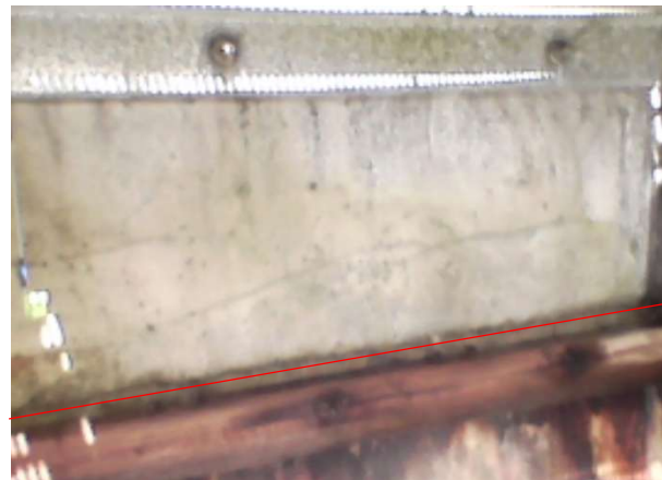
Bay 12 – Looking west
