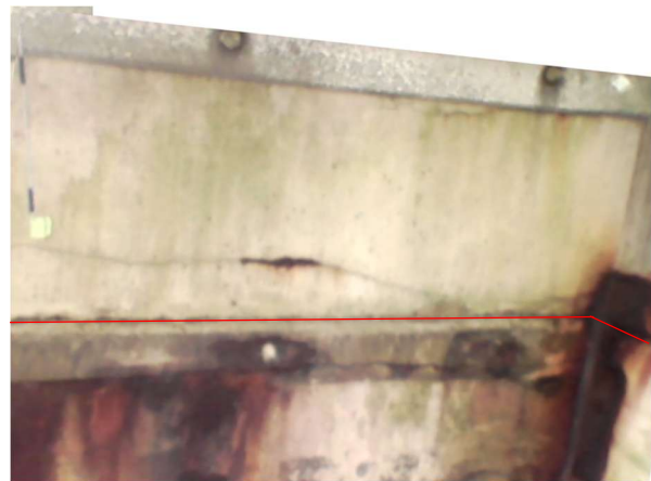
Bay 17 - Looking east
