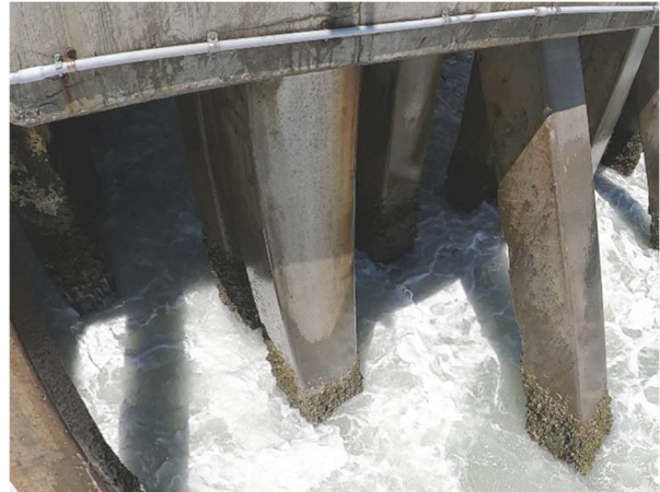
Armor stone inside the crib near low tide
