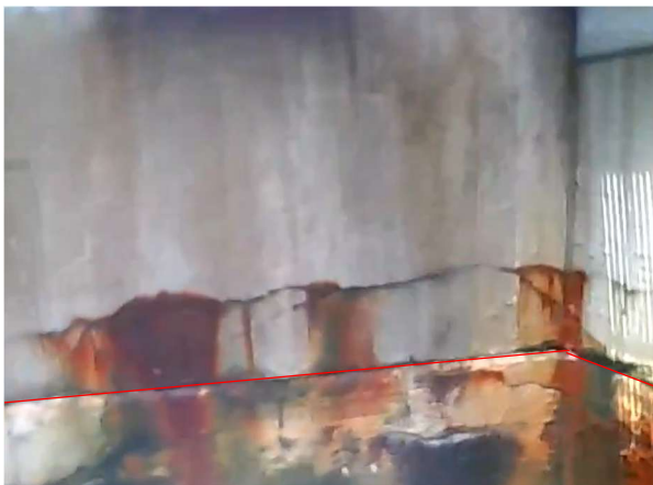
Bay 42 – Looking south
