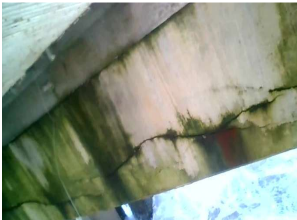
Bay 57 - Looking East
