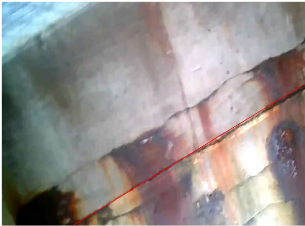
Bay 44 - Looking South
