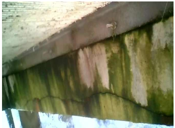
Bay 56 - Looking East
