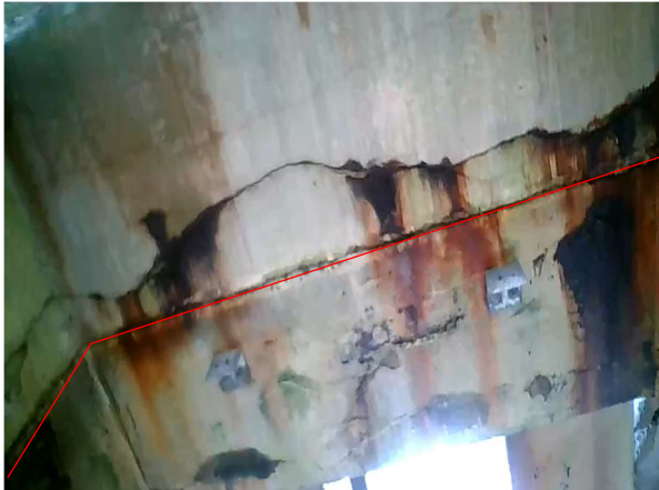
Bay 36 – Looking South
