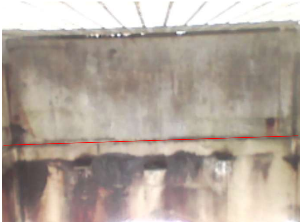
Bay 25 – Looking north
