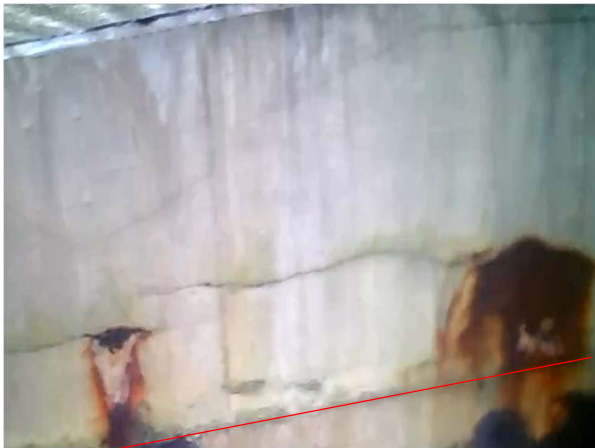
Bay 8 – Looking south
