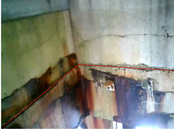
Bay 23 – Looking east
