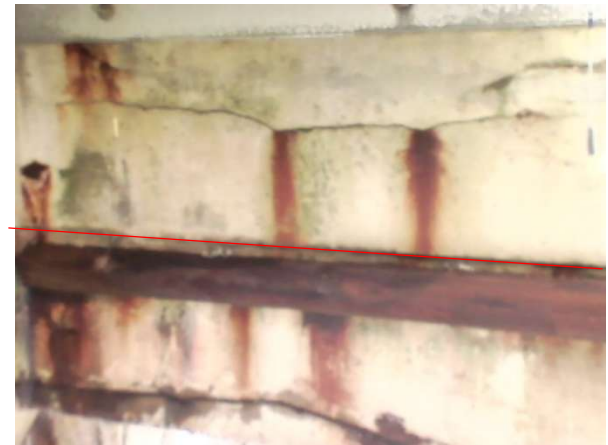
Bay 27 – Looking West
