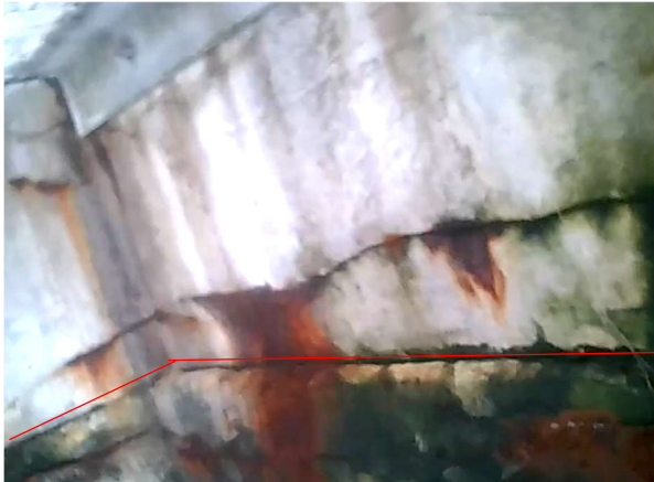
Bay 55 - Looking East
