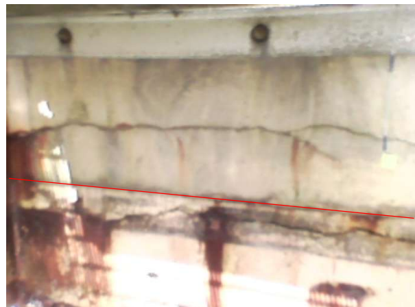
Bay 9 – Looking west
