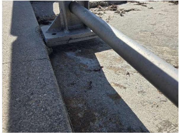
Unsupported intermediate post base plate
