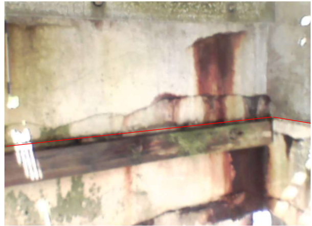
Bay 21 – Looking west
