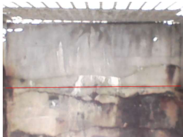
Bay 7 - Looking North
