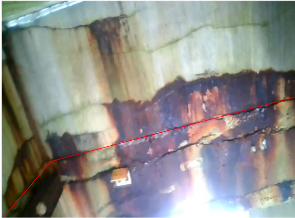
Bay 33 – Looking South
