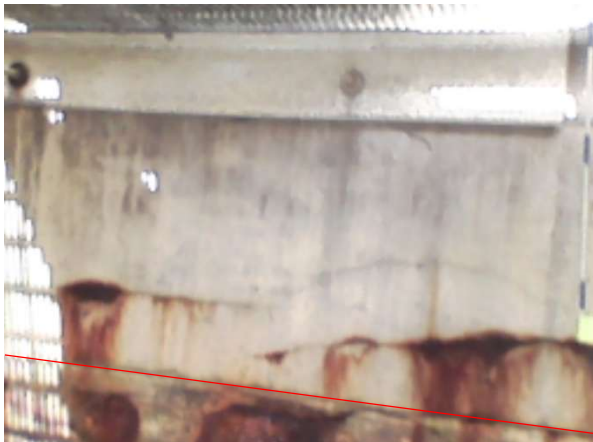
Bay 2 – Looking West
