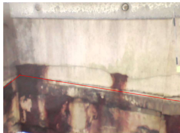
Bay 17 - Looking west
