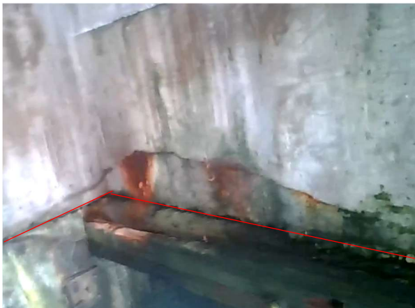
Bay 54 - Looking East
