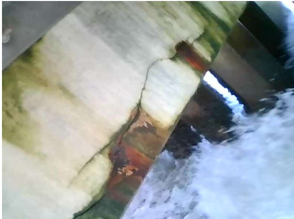
Bay 58- Looking West
