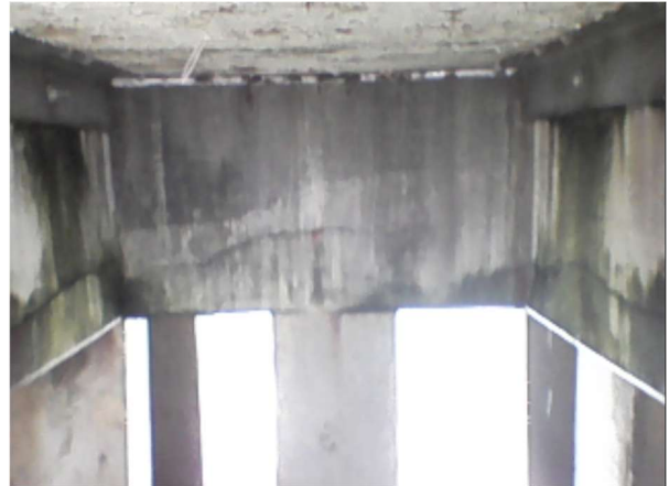
Bay 58- Looking North
