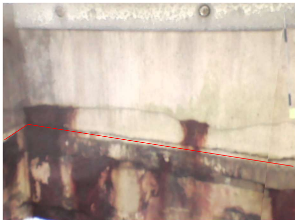
Bay 17 - Looking east
