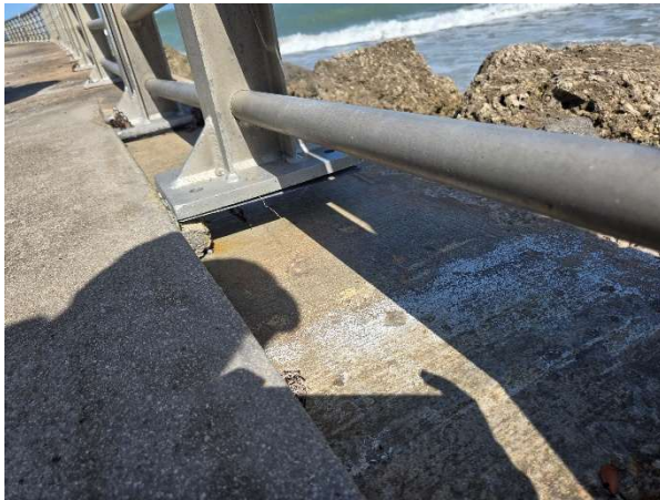
Unsupported intermediate post base plate
