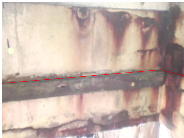
Bay 27 – Looking East
