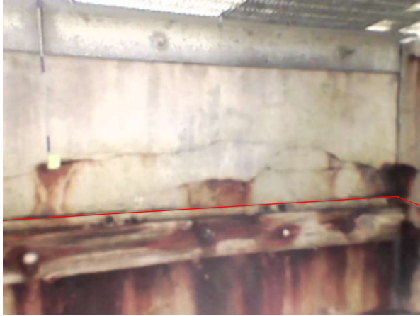
Bay 3 – Looking West
