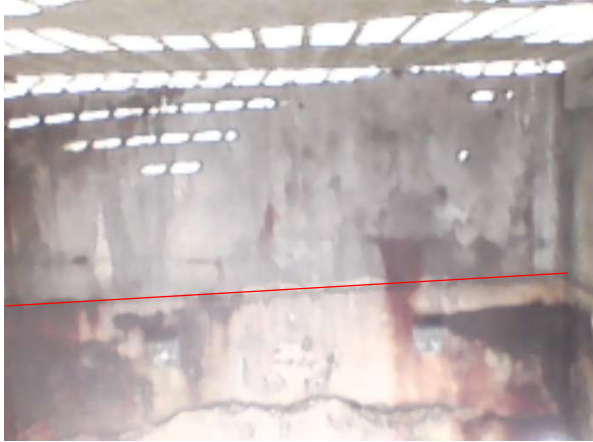
Bay 10 – Looking north
