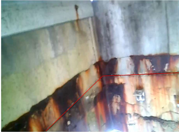
Bay 25 - Looking southeast
