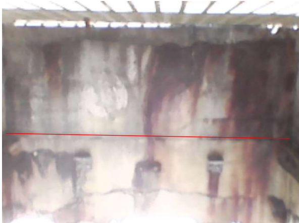
Bay 12 – Looking north
