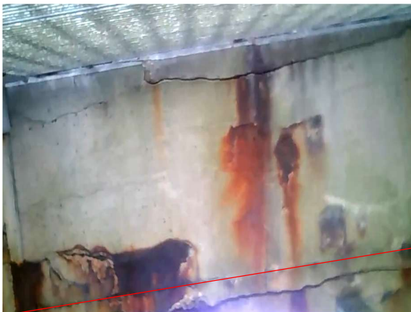
Bay 6 – Looking South
