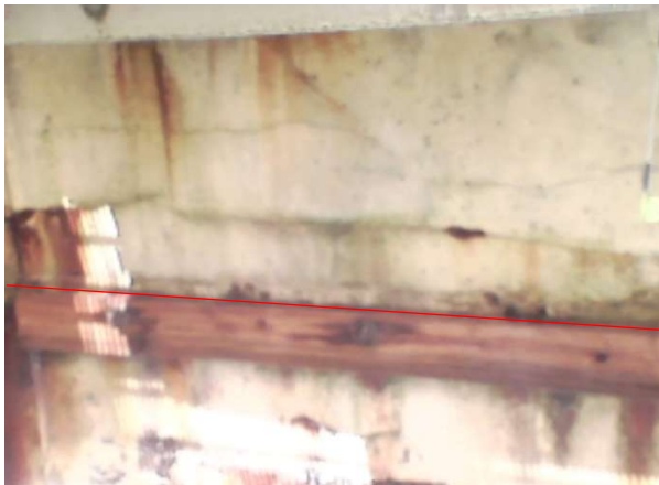
Bay 12 – Looking west
