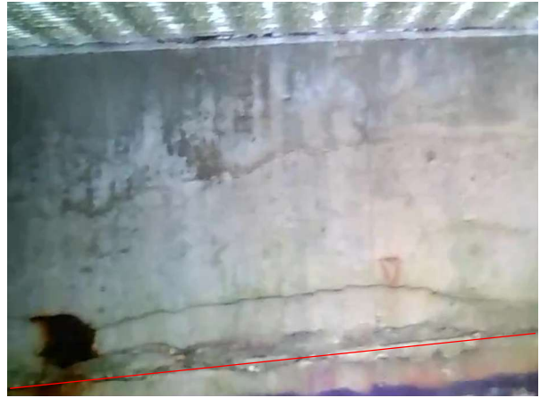
Bay 5 - Looking South
