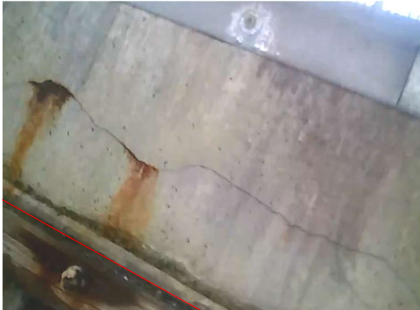
Bay 2 - Looking East
