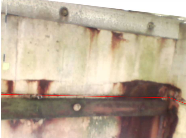
Bay 21 – Looking east
