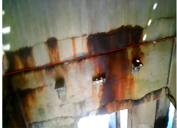
Bay 34 – Looking North
