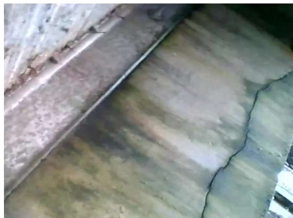
Bay 58- Looking East
