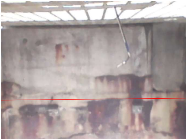
Bay 18 - Looking north
