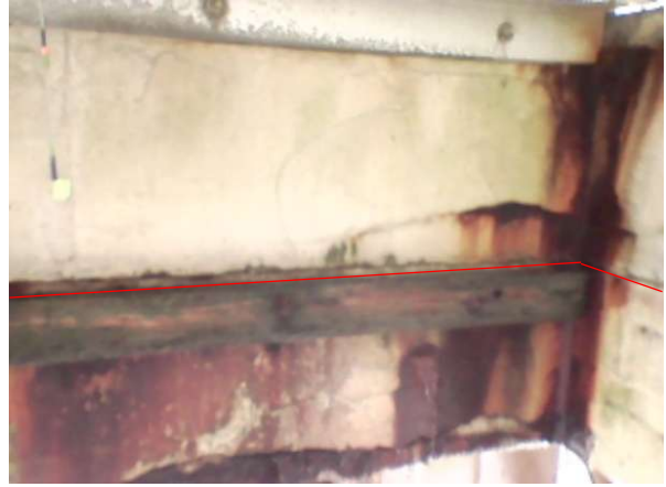
Bay 30 – Looking East
