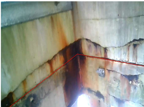
Bay 36 – Looking East
