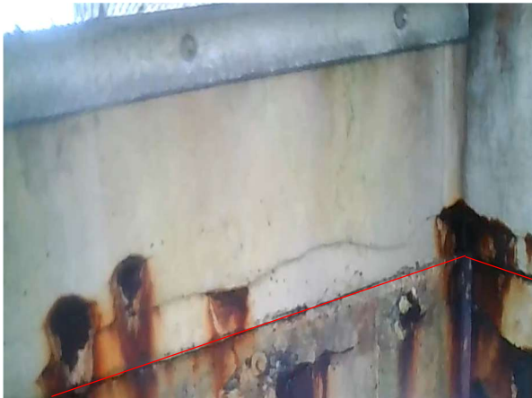
Bay 39 – Looking East
