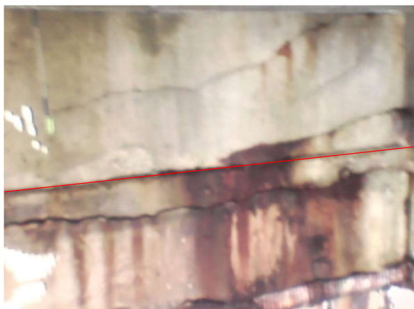
Bay 17 - Looking west
