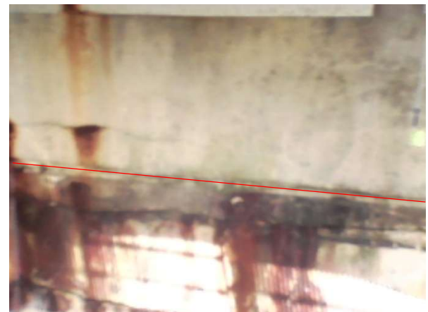
Bay 11 – Looking west
