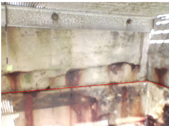
Bay 14 – Looking east
