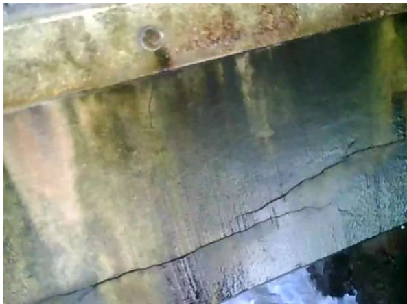
Bay 59- Looking West
