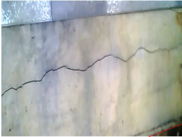
Bay 4 - Looking East
