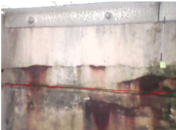
Bay 1 – Looking East
