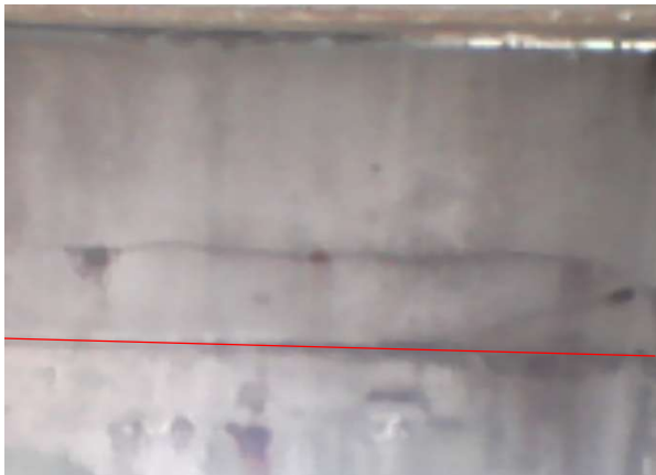
Bay 1 – Looking North
