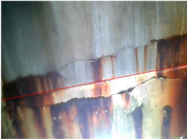
Bay 41 – Looking South
