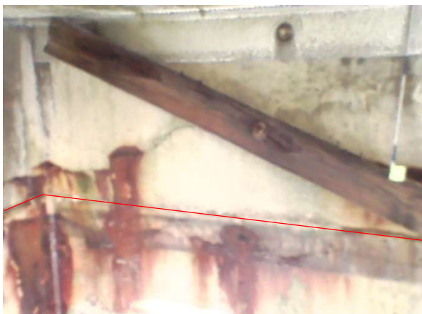
Bay 13 – Looking west
