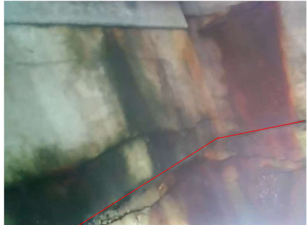
Bay 55 - Looking Southeast
