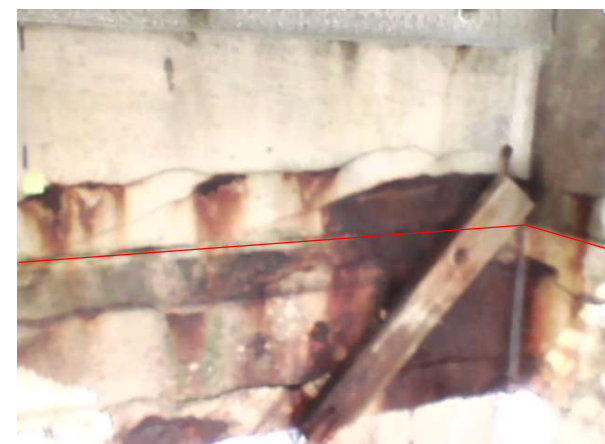
Bay 20 – Looking west
