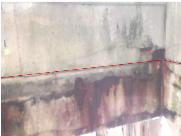
Bay 18 - Looking east
