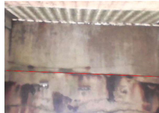
Bay 1 – Looking South
