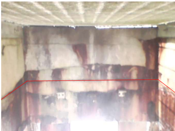
Bay 31 - Looking South
