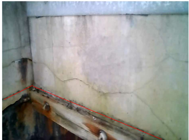
Bay 7 - Looking East
