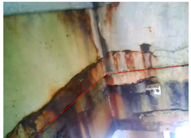
Bay 22 – Looking east
