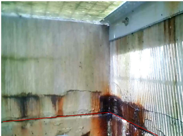
Bay 37 - Looking Southwest
