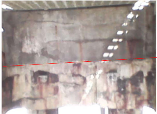
Bay 19 - Looking north
