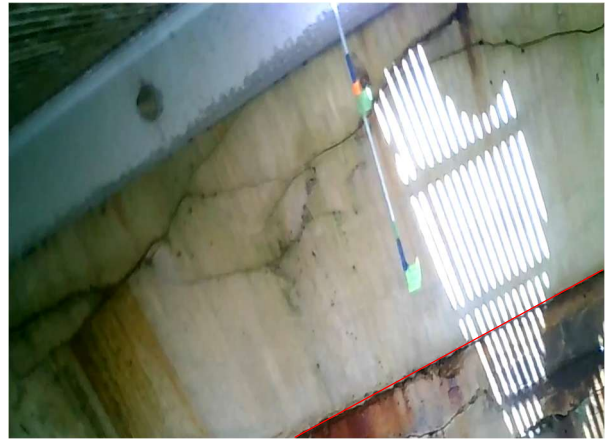
Bay 33 – Looking West
