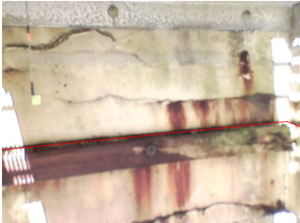
Bay 27 – Looking west
