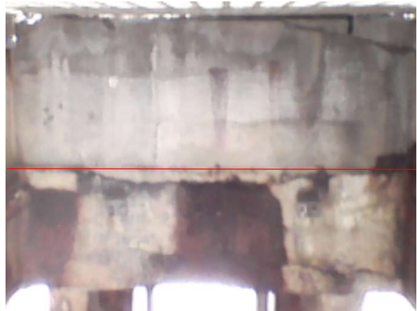
Bay 6 – Looking north
