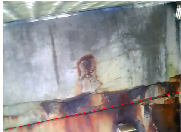
Bay 13 – Looking south
