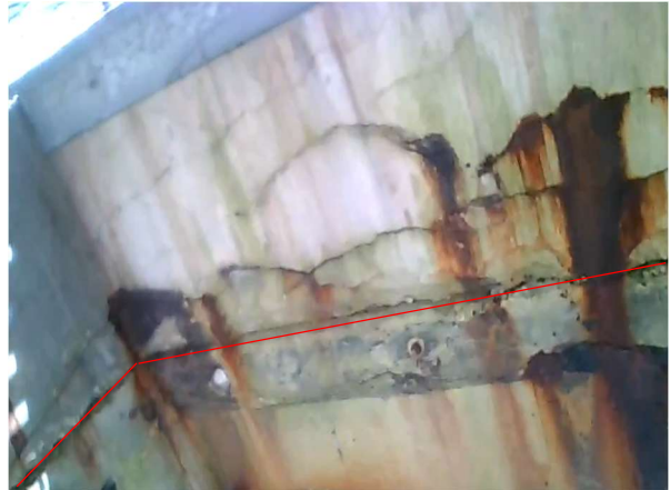
Bay 36 – Looking East
