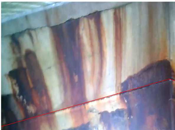
Bay 40 - Looking South
