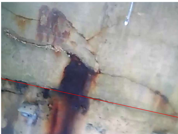
Bay 3 – Looking South
