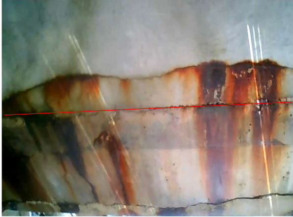
Bay 51 - Looking West
