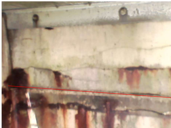
Bay 19 - Looking west
