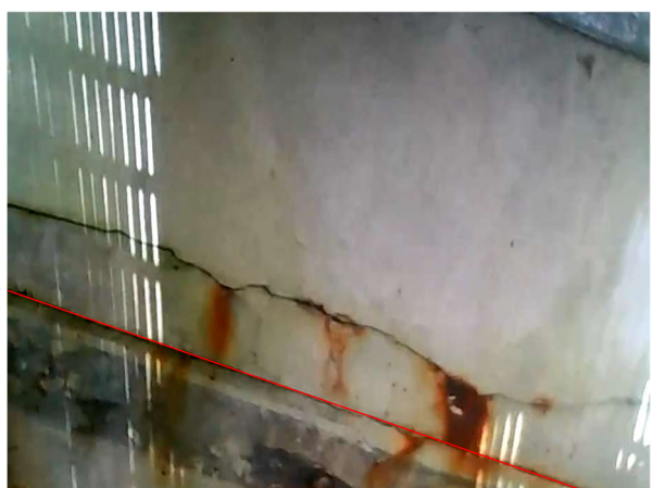
Bay 3 – Looking West
