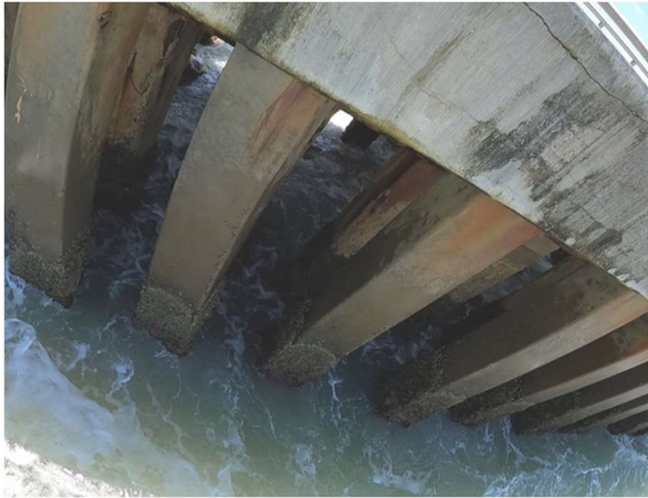
Armor stone inside the crib near low tide
