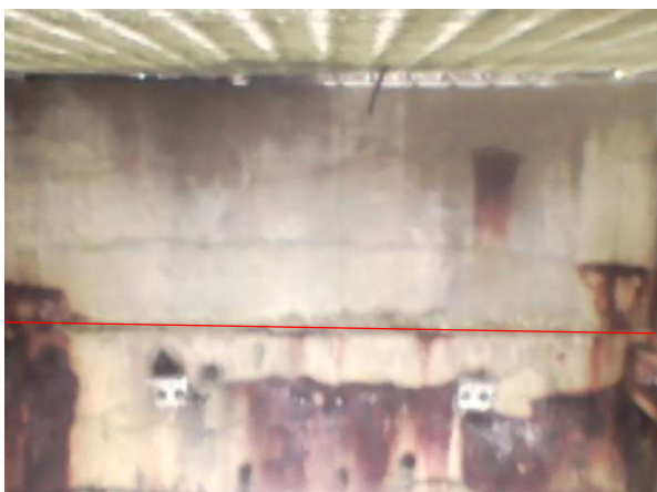
Bay 21 – Looking north
