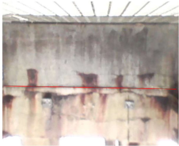
Bay 26 – Looking north
