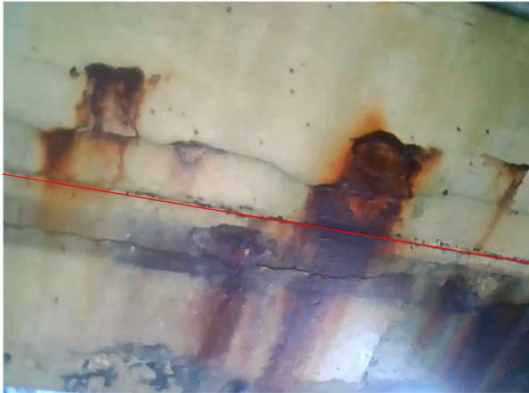
Bay 45 - Looking East
