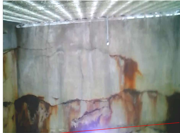
Bay 4 - Looking South
