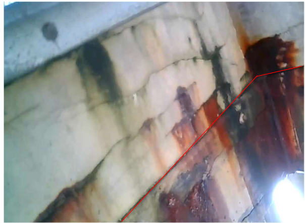
Bay 44 – Looking East
