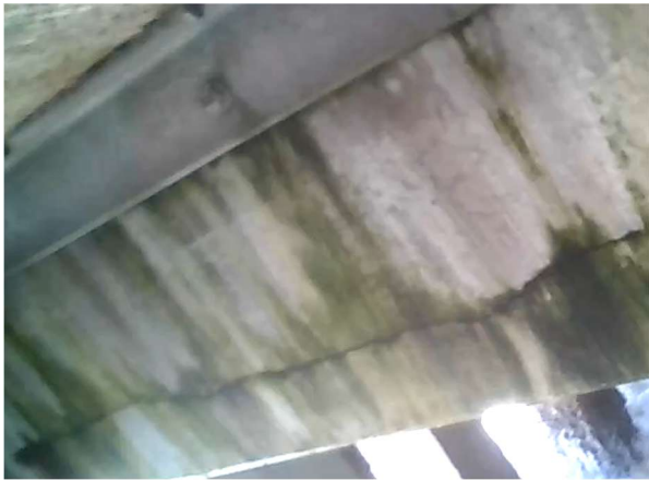
Bay 57 - Looking West
