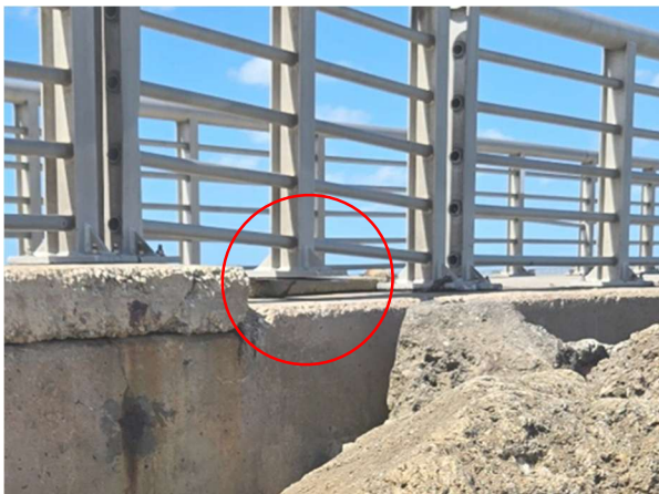
Unsupported intermediate post base plate
