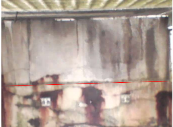
Bay 18 - Looking south
