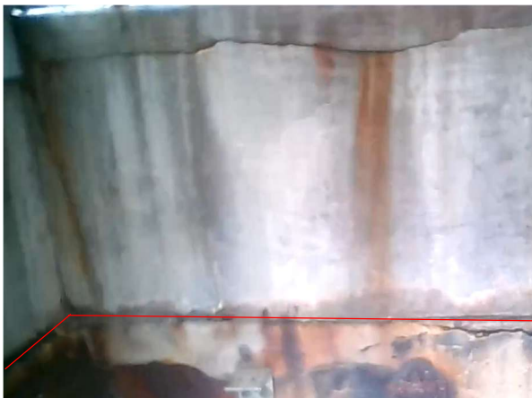
Bay 49 - Looking South
