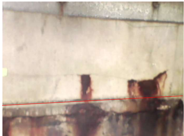
Bay 8 – Looking east
