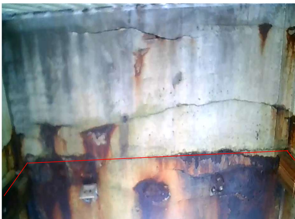
Bay 12 - Looking south
