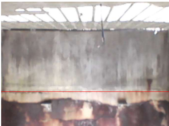
Bay 16 – Looking north
