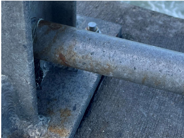
Railing corrosion
