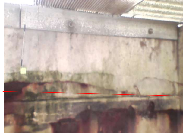
Bay 1 – Looking East
