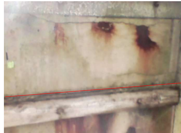
Bay 14 – Looking east
