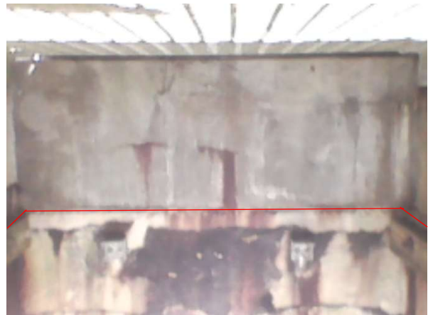
Bay 21 – Looking north
