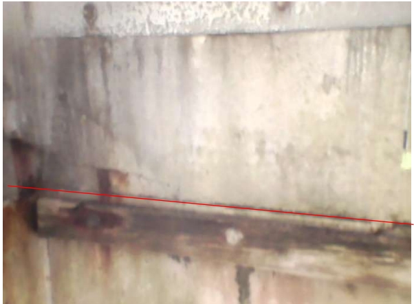
Bay 13 – Looking east
