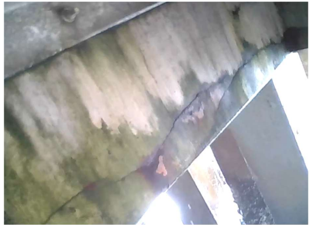
Bay 57 - Looking East
