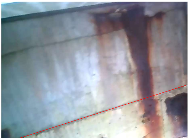
Bay 40 – Looking North
