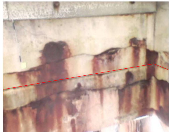
Bay 6 – Looking East
