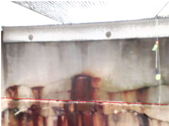
Bay 48 - Looking West
