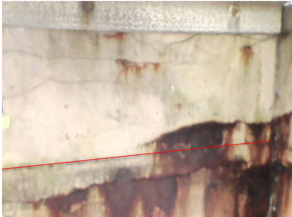
Bay 10 – Looking east
