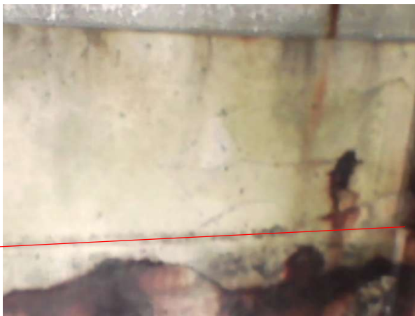
Bay 9 – Looking east
