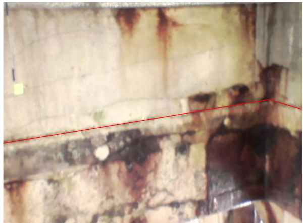
Bay 19 - Looking east
