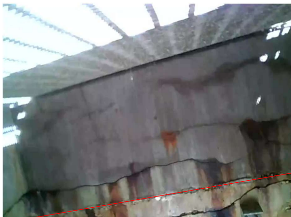
Bay 17 - Looking north
