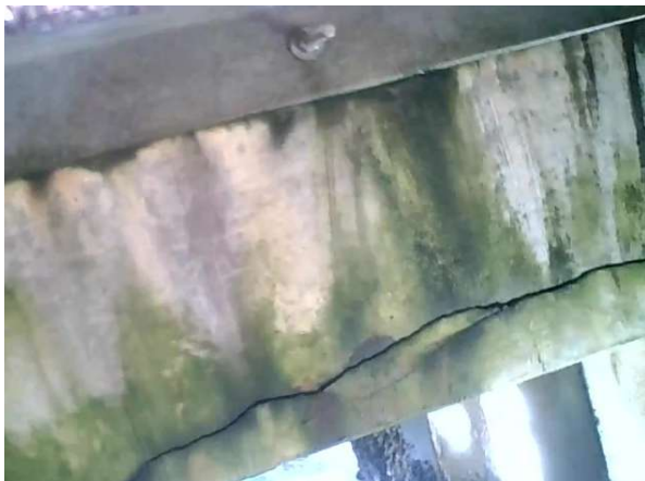
Bay 56 - Looking East
