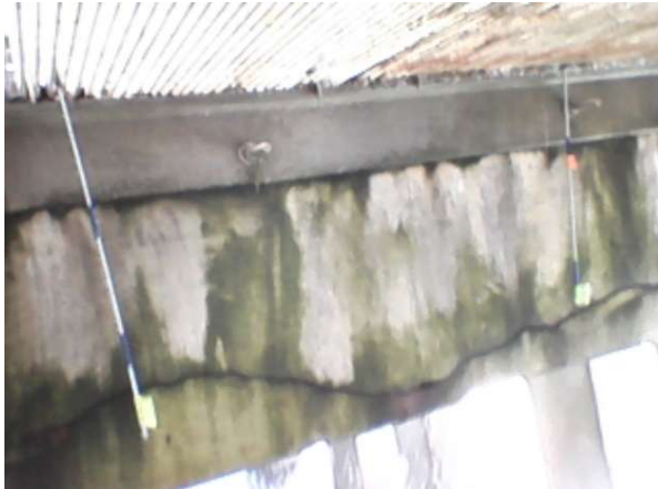
Bay 58- Looking East
