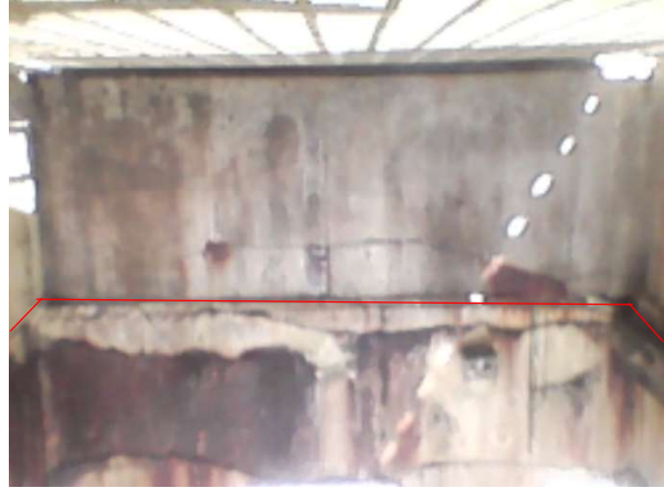
Bay 23 – Looking north
