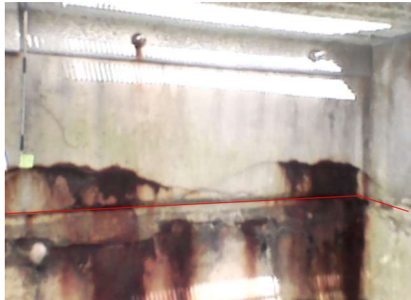
Bay 2 – Looking West
