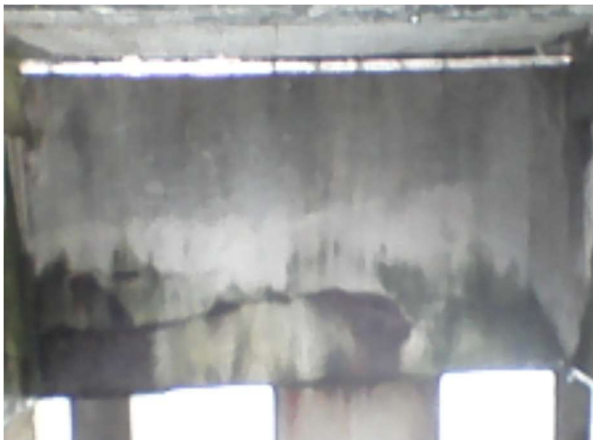
Bay 59- Looking West
