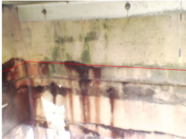
Bay 26 – Looking east
