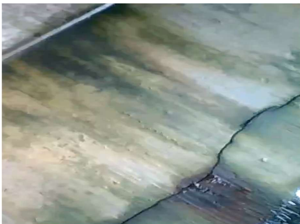
Bay 58- Looking East
