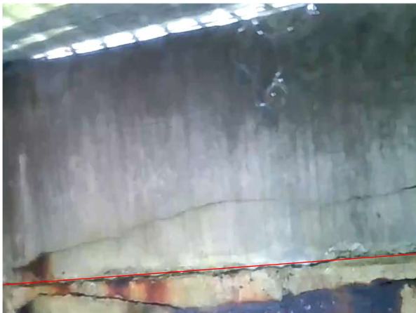
Bay 16 – Looking South
