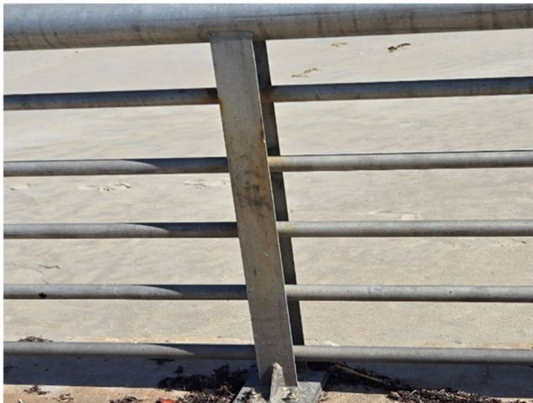
Railing corrosion
