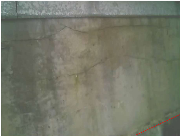
Bay 5 - Looking East
