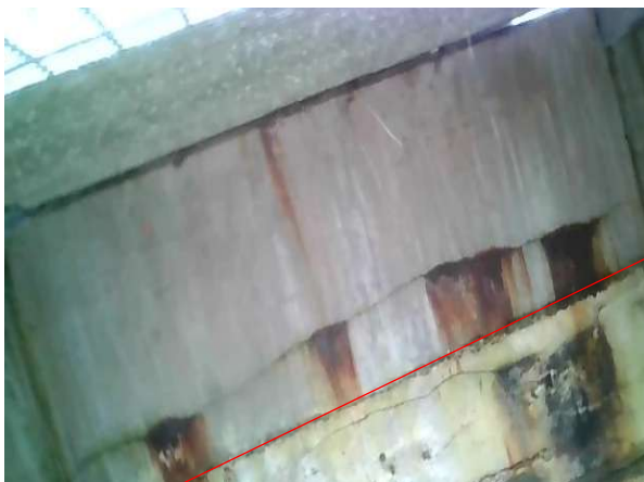
Bay 38 - Looking North
