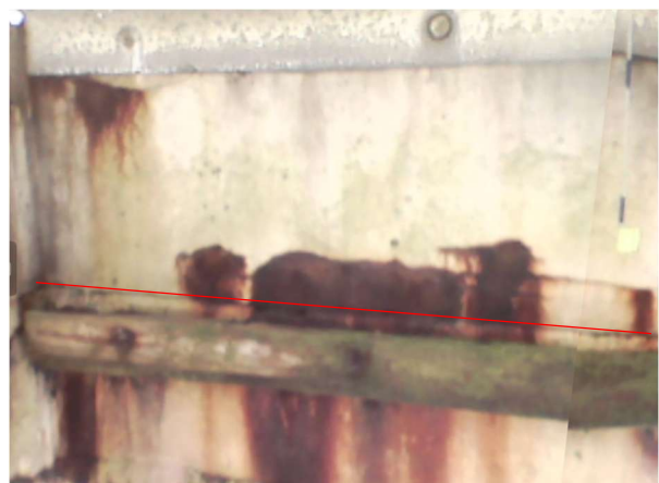
Bay 21 – Looking east
