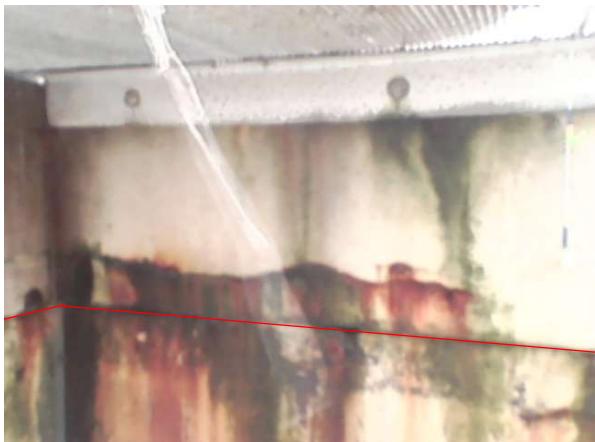
Bay 44 - Looking West
