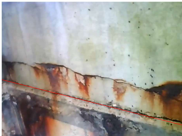
Bay 20 - Looking east
