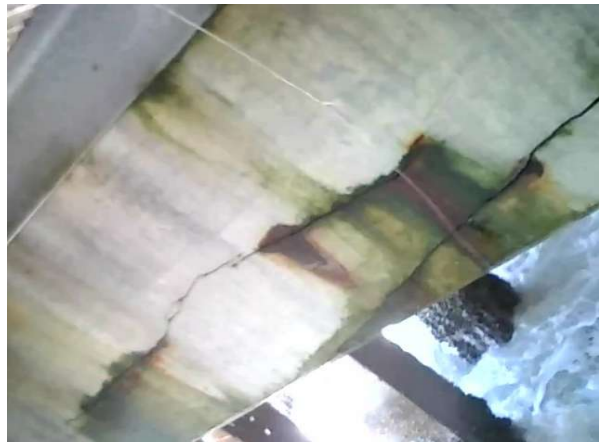
Bay 58- Looking West
