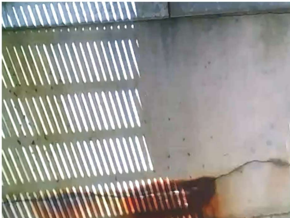
Bay 7 - Looking West
