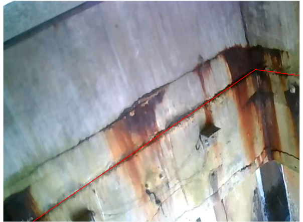
Bay 35 – Looking North
