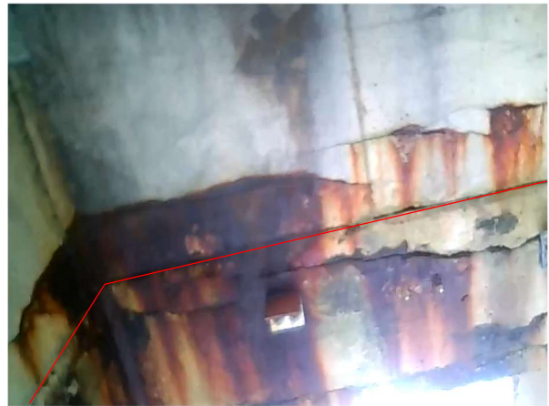
Bay 28 – Looking south
