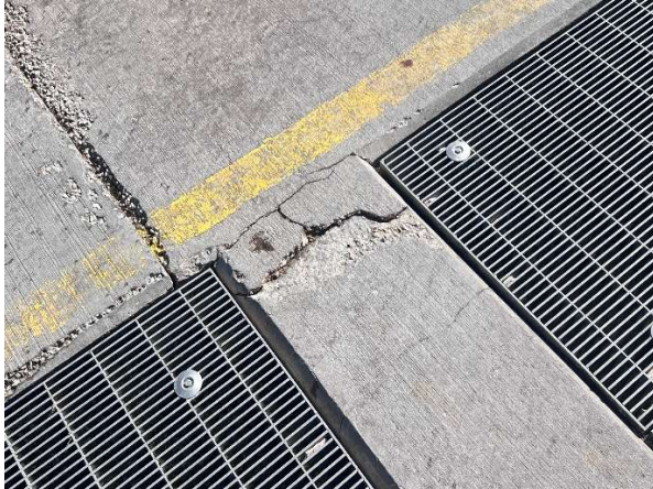
Spall at top of pile cap, Bay 30
