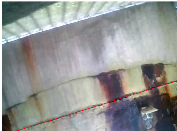
Bay 17 - Looking south
