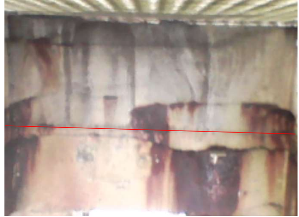
Bay 10 – Looking south
