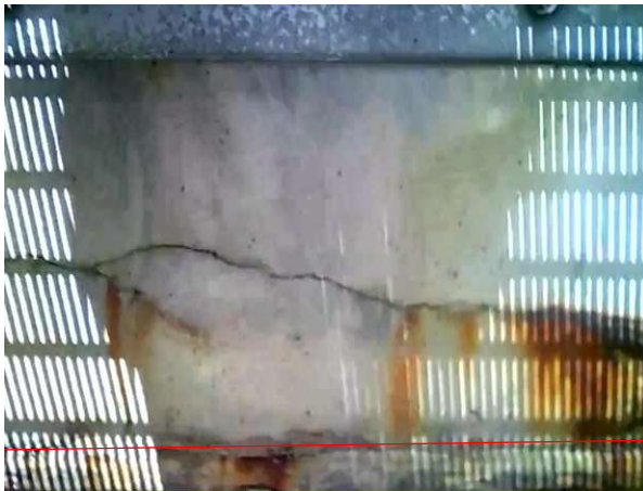
Bay 9 – Looking west
