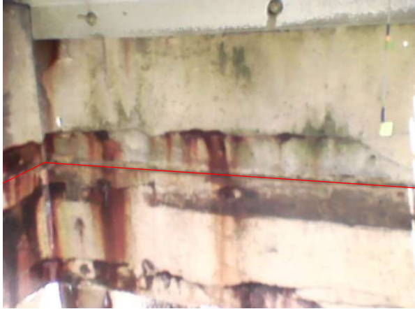
Bay 30 – Looking West
