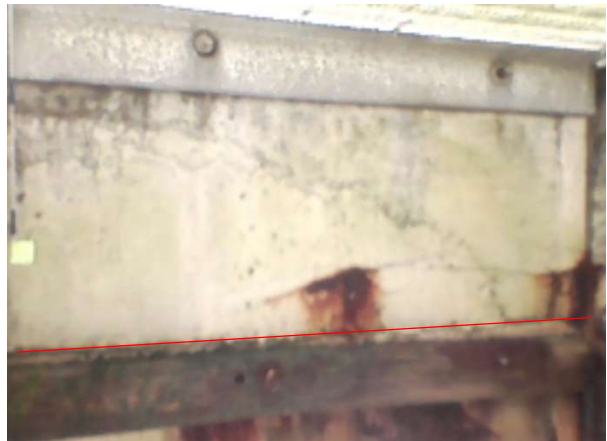
Bay 12 – Looking east
