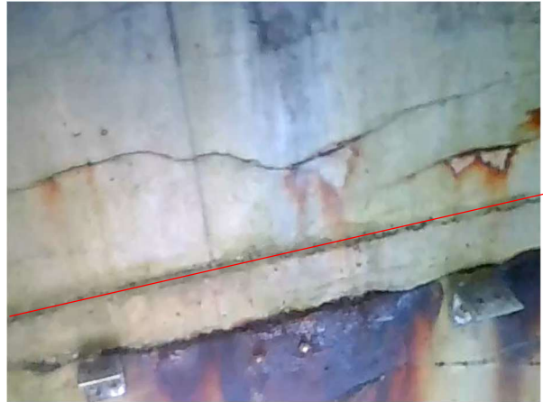
Bay 14 – Looking south
