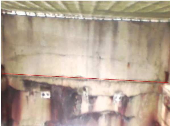
Bay 23 – Looking south
