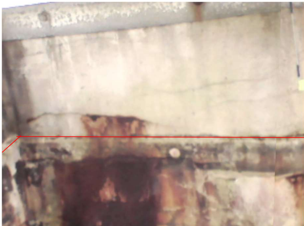
Bay 19 - Looking east
